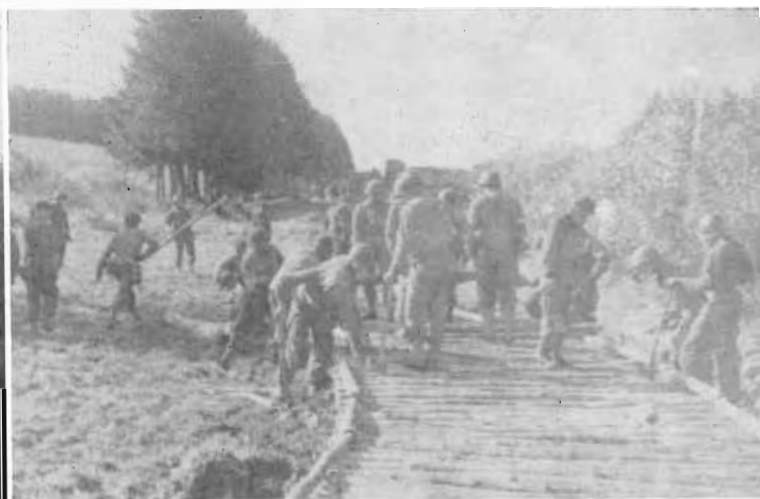
Corduroy road near Houffalize, Belgium, is built by Fourth Engineers to aid our drive on the Siegfried Line. September 1944.
