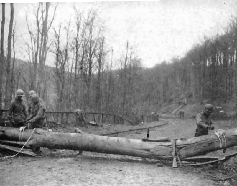
This is one way of removing logs from the road, TNT charges, road east of Prum, Germany, March 2, 1945.
