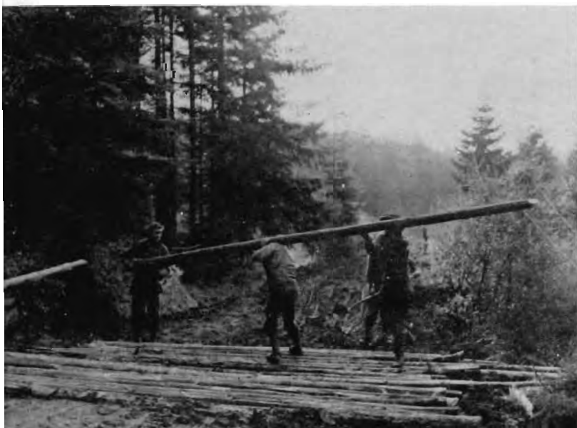
Another corduroy road is built by the engineers through the areas of the Hurtgen Forest. November 1944.
