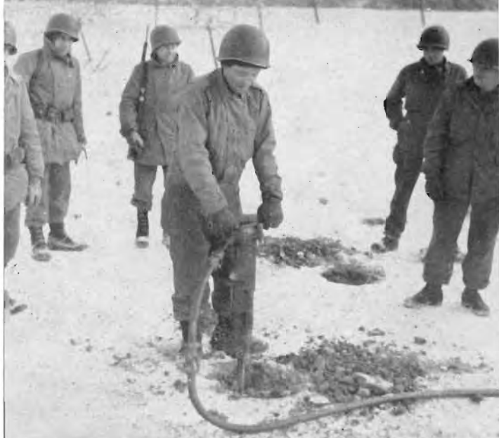
Supporting engineers drill holes for mines to be placed as protection against German armor. January, 1945, Luxembourg.
