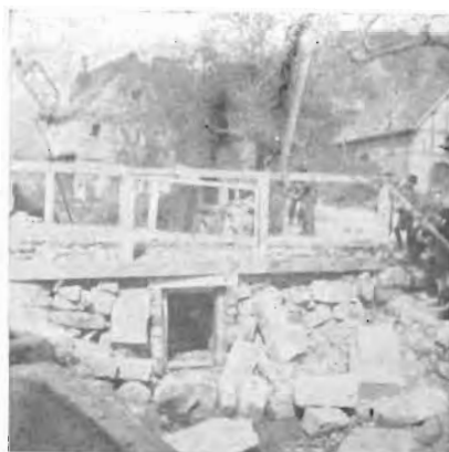
Culvert constructed by Fourth Engineer Battalion north of Rothenburg.
